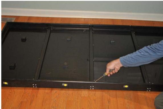
8. Then finally use the two remaining “Module Attaching Screws” to attach the Left Center Module to the Left Module.
