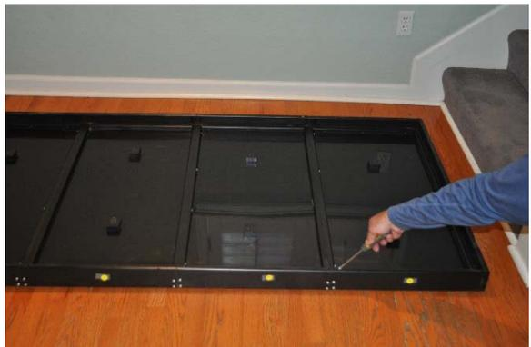
7. In a similar fashion, use two “Module Attaching Screws” to attach the back and front of the Left Center Module to the Right Center Module.
