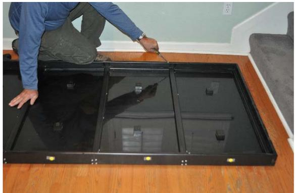
6. Then using a second “Module Attaching Screw”, attach the front side of the Right Center module to the front side of the Right Module.
