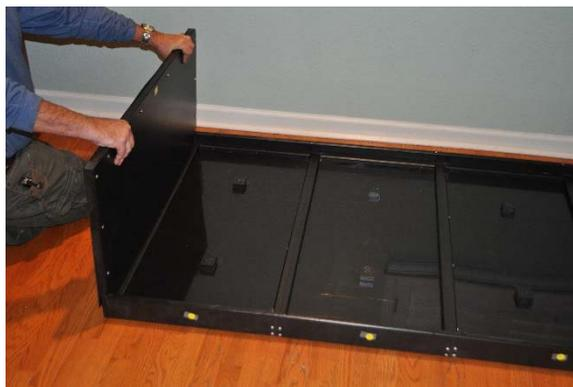
12. While holding this panel in place, slide “Panel 2” onto the left half of the back side of the box frame.
