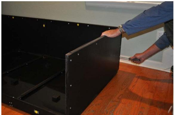
18. Using the “Base Screws” provided, attach the bottom of each of the polyethylene panels to the box frame using the pre-drilled screw holes. There are two screws for each panel.
